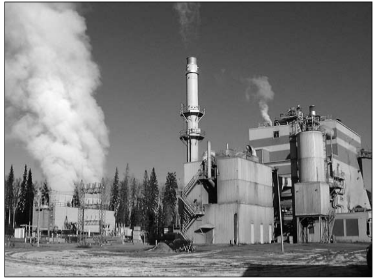
Above and right: the 23MW Whitecourt biomass project in Alberta.
