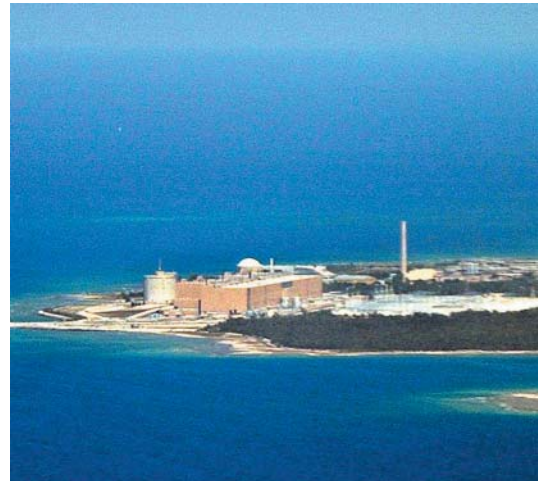
Bruce Nuclear Station. The return to service of Bruce Power's Units 3 and 4 and OPG's Pickering Unit 4 have significantly improved Ontario's electricity supply.
